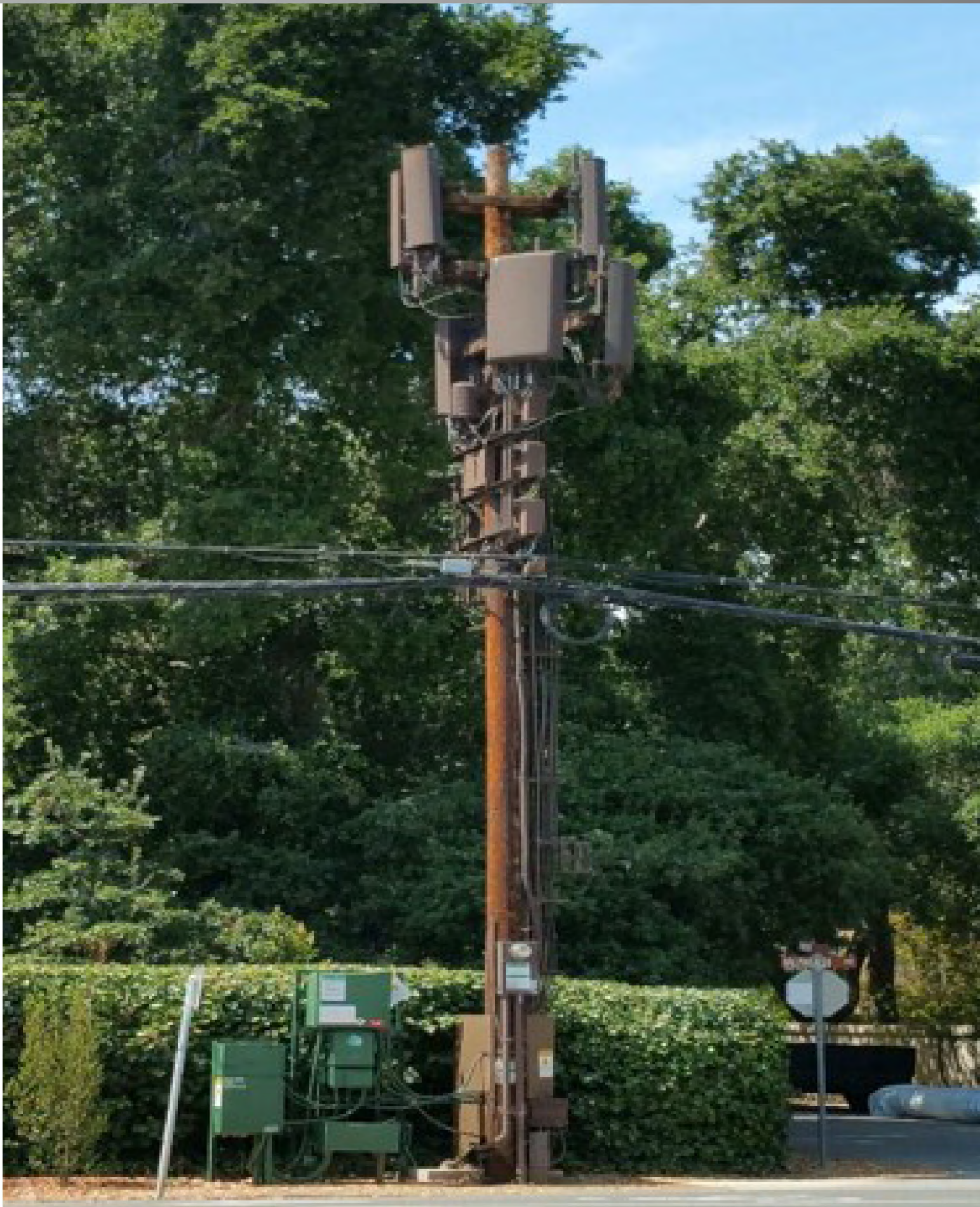
Example of a cluttered small cell install
